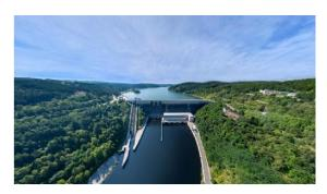
The Orlík dam is a main element of the chain of dams on the Vltava river. With its capacity of 720 million m³ of water, it is the largest reservoir in the Czech Republic, and together with the Lipno Lake (southward in the Šumava area) it is crucial for water-flow control on both the Vltava and the lower Elbe. A secondary effect is the electric power generation, especially during peak hours.
